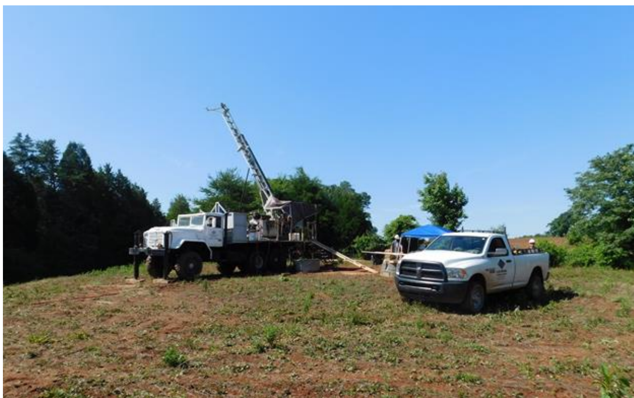
Figure 2: Phase 2 Drill Rig On-Site
